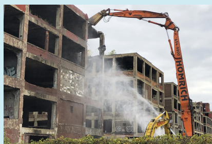
Packard Plant Undergoing Demolition
